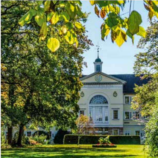
The Kurhaus Bad Boll
