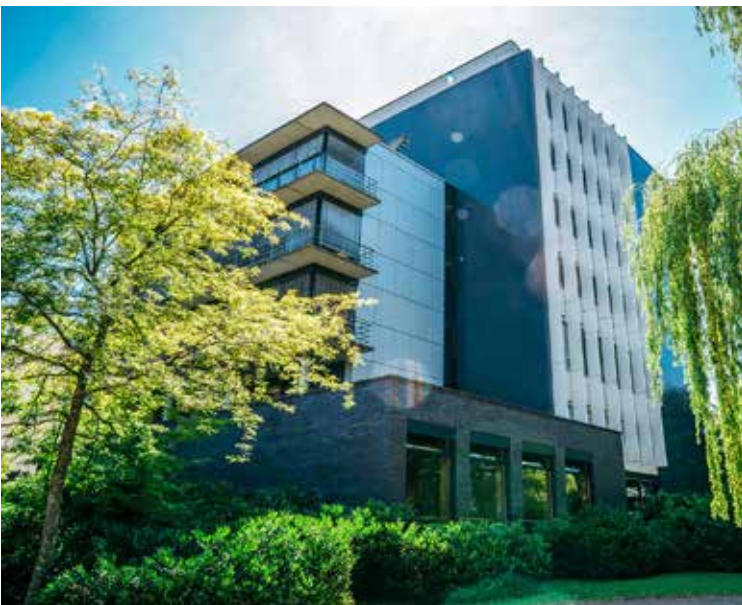
Building Pa4 of the HfWU in Geislingen
