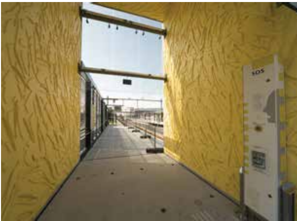
The concrete design of a Dutch subway line based on the template designed by the designer Erik Sandifor from Rotterdam
