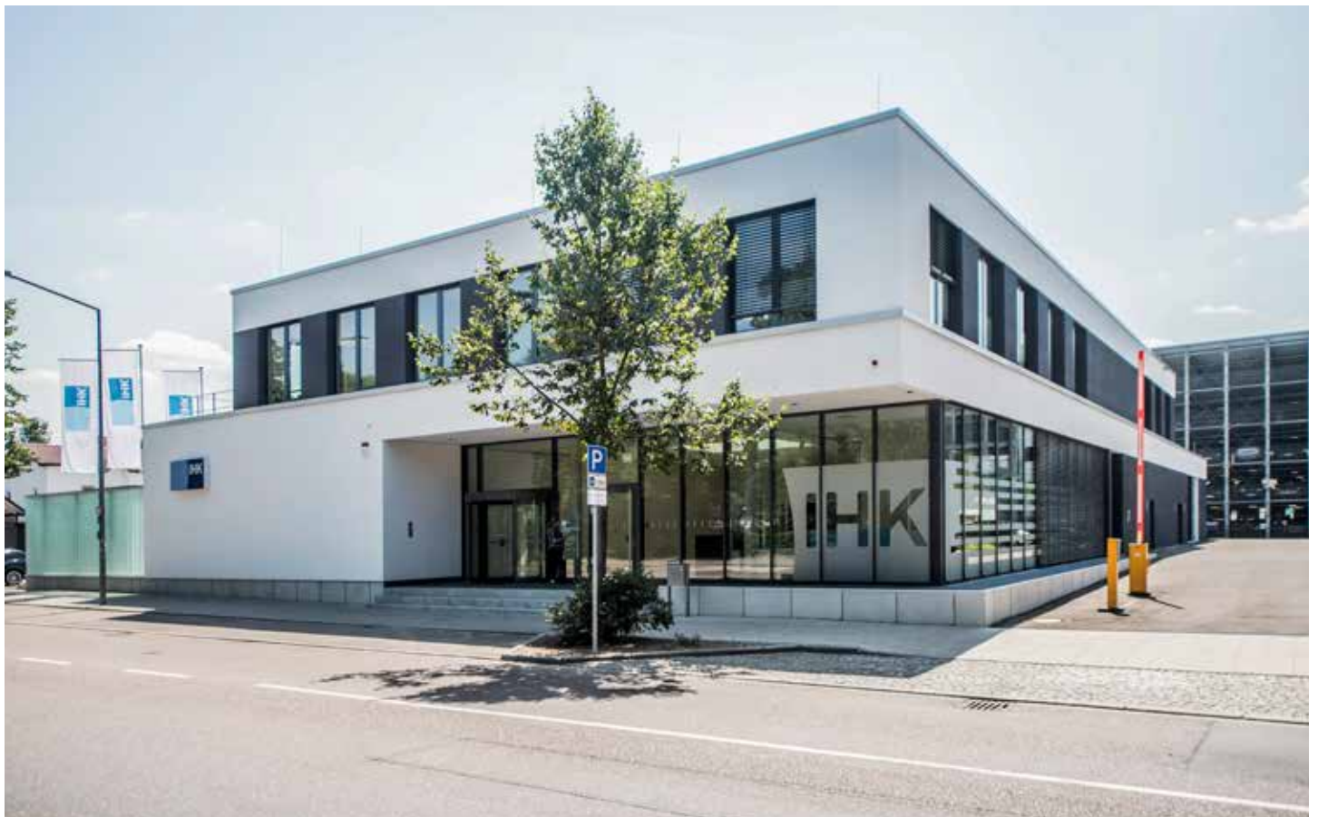
The Chamber of Industry and Commerce at the Göppingen business location
